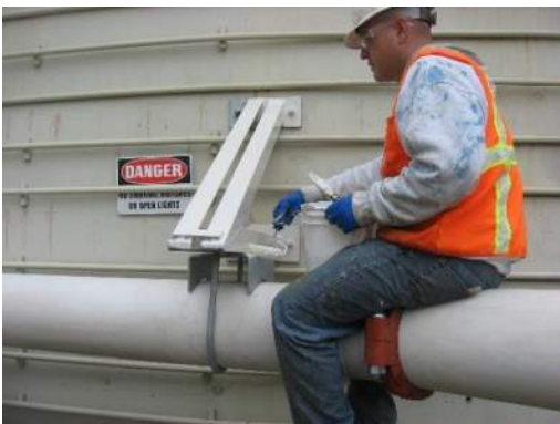
Photo 4-23. Application with rollers and brushes.
