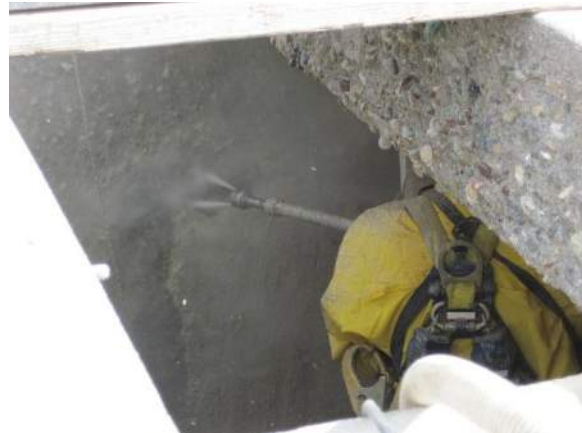
Photo 4-22. Ultra high pressure water jetting on a concrete structure.
