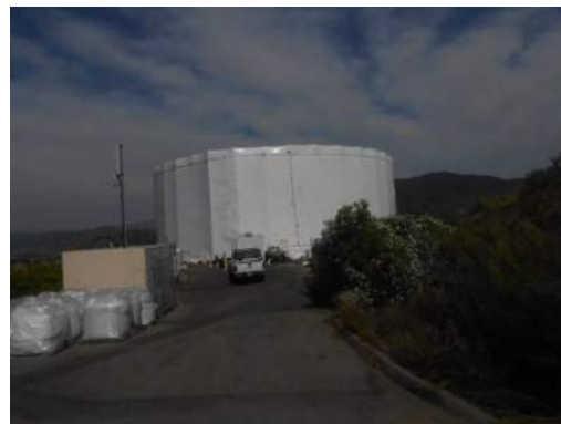
Photo 4-24. Full containment is required for abrasive blasting.
